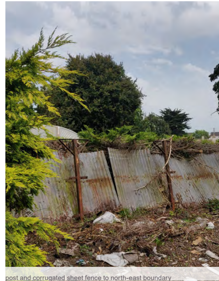
post and corrugated sheet fence to north-east boundary
