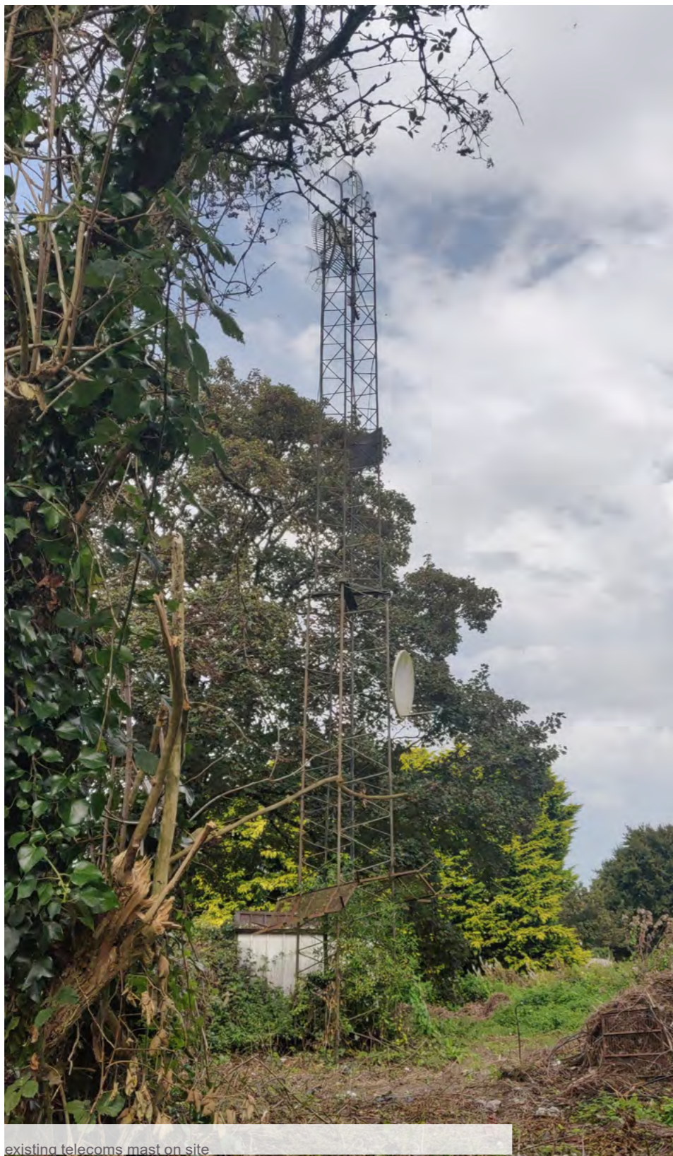
existing telecoms mast on site
