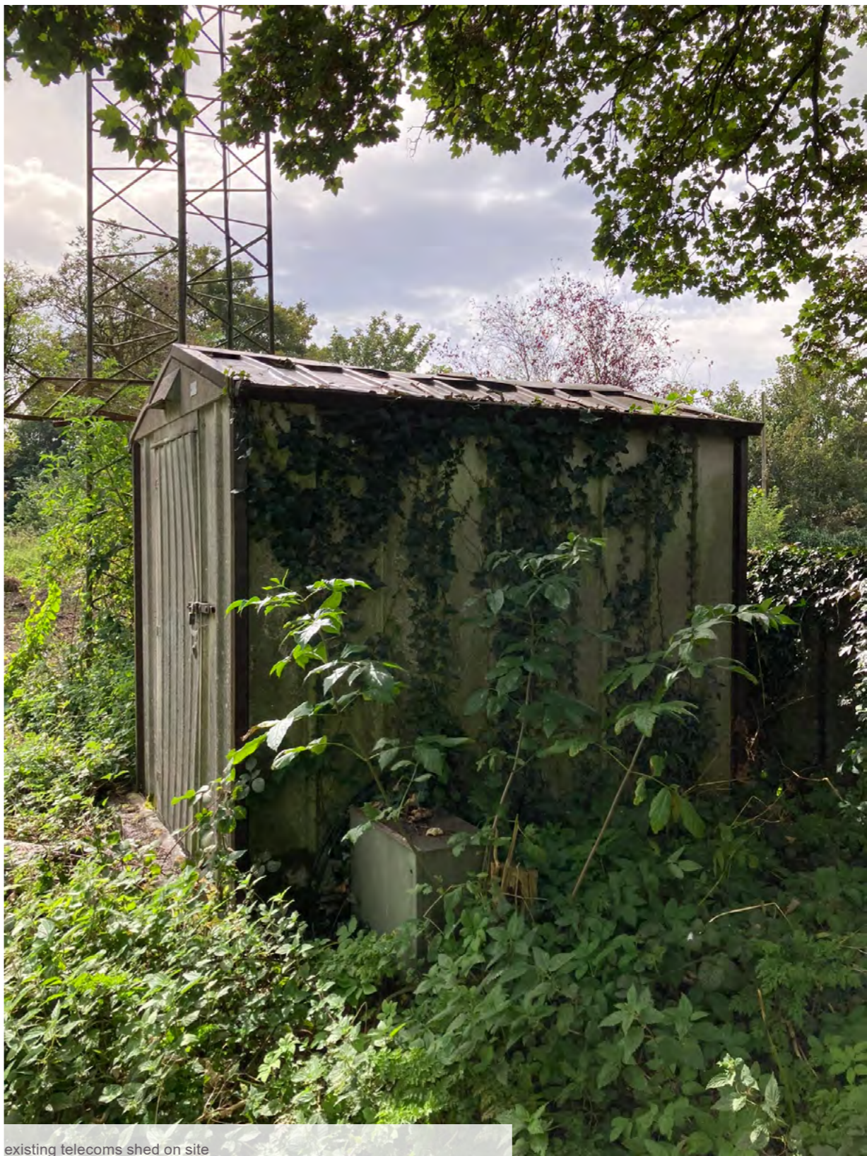
existing telecoms shed on site
