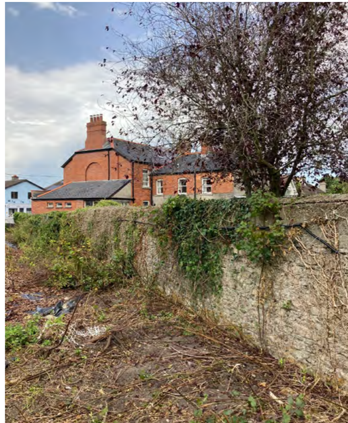
stone and concrete wall to north boundary adjacent site entrance
