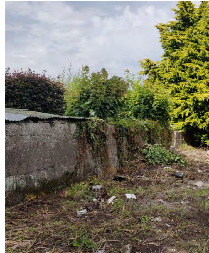
concrete wall to north-west boundary
